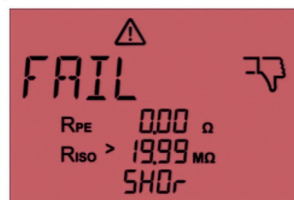
Fig. 48: Failed measurement. "SHOr" is shown on the display. Short circuit between L and N
